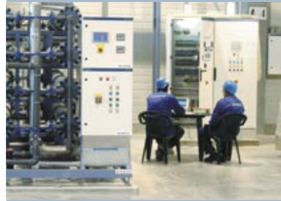
Preventive service of water treatment plant at car manufacturer.
