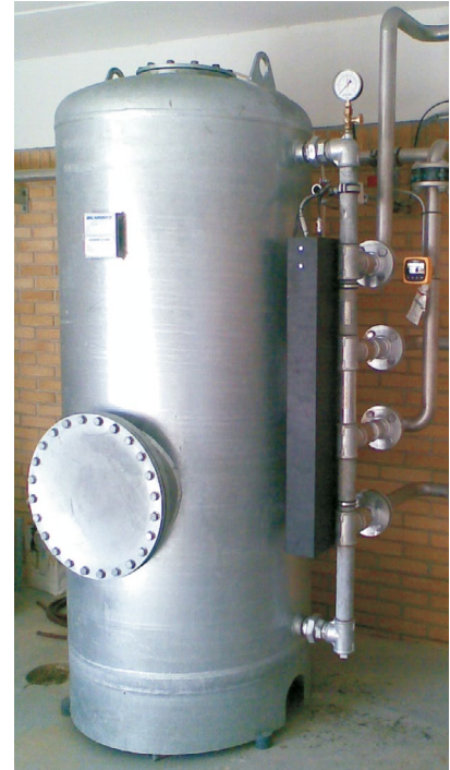
Arsenic removal by means of adsorption in waterworks. The solution comprises an automatic pressure filter type NSB 170 installed after open filters. Flow rate: 12 m 3 /h.
