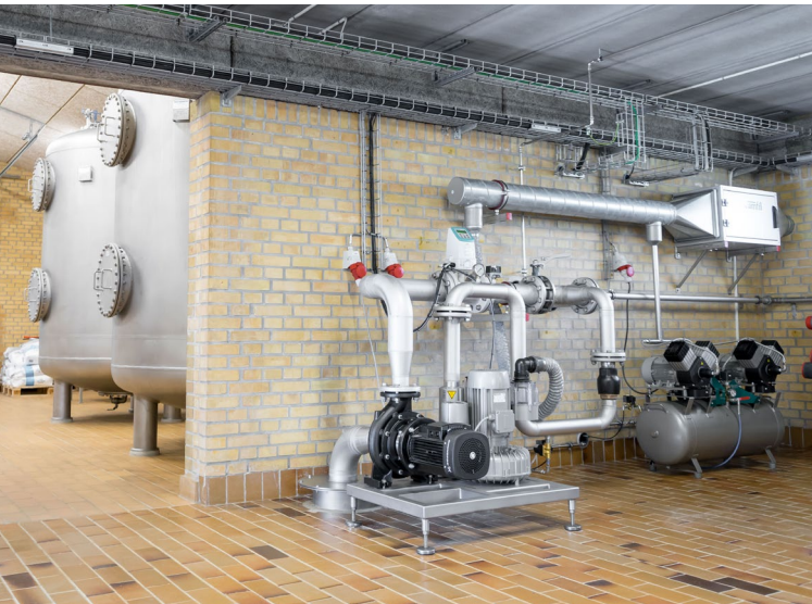
Complete water treatment solution comprising a stainless steel pressure filter and technical equipment for oxidation and backwashing.
