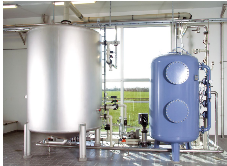
Degassing of dissolved gases such as aggressive carbon dioxide, methane, and hydrogen sulphide is a precondition of optimum filtration. Photo: Degassing and surface coated pressure filter in brewery.
